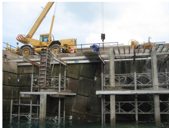
Works in progress
